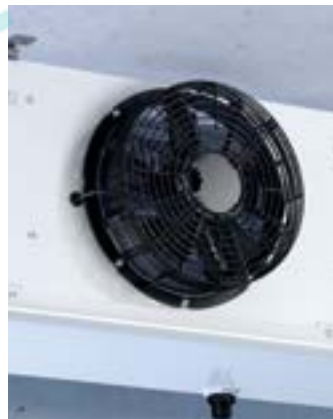
SP 23 = ESM-Motor [EC Technology]
