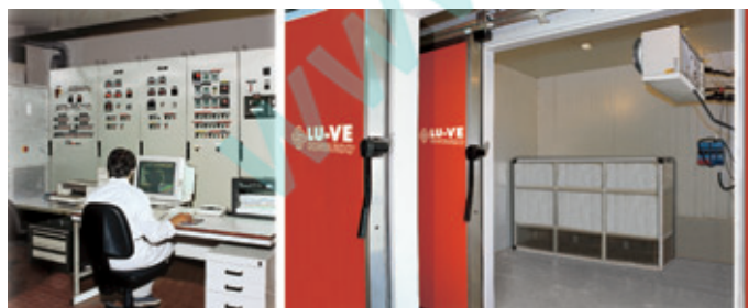
Dooble cold rooms laboratory
